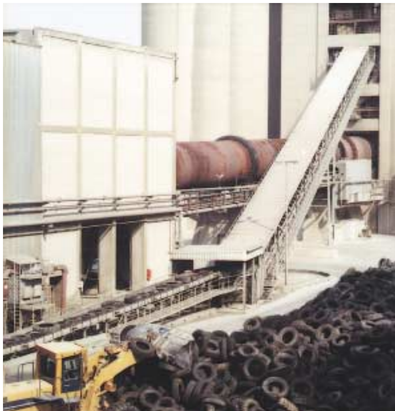
Worn tires being fed into the rotary tubular kiln
